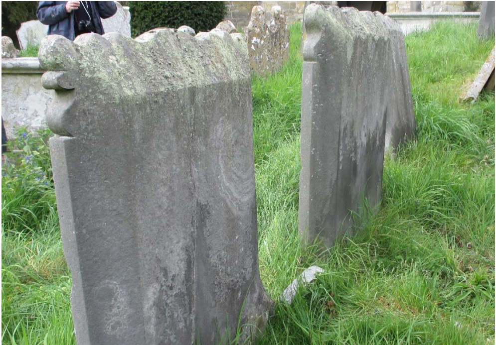
The rear of the same headstones showing the chamfered edge at the top of the headstone.
